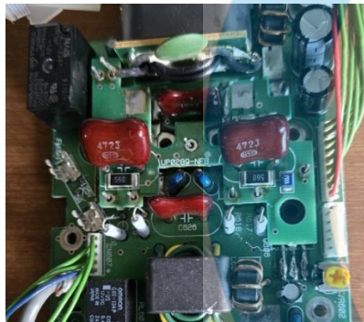
Figure 4 - Repaired daughterboard in place in radio – not yet soldered in
