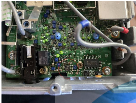
Figure 3 - IC151 location on RF UNIT board
