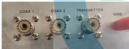
Figure 4 - re-mounted SO-239 jacks
