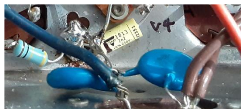
Figure 9 - Safety capacitors installed at power entry point
