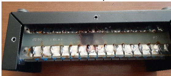
Figure 2 - Charred spot on PCB
