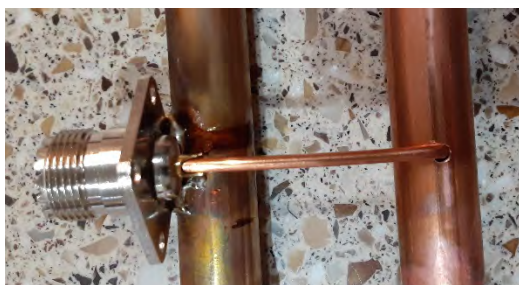
Figure 14 - 10AWG wire in place
