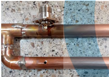
Figure 13 - Hole for wire drilled
